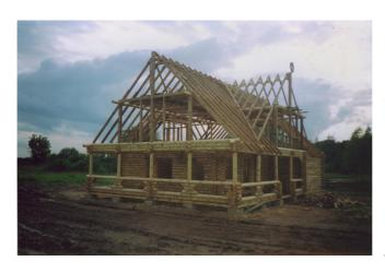
planed. Afterwards – at least 4 months of ventilating After draughty premises. ventilating timber is considered qualitative. logs are dried and ready houses don't crack after construction. It is necessary to prepare 300 - 400 m<sup>3</sup> of timber for work in
